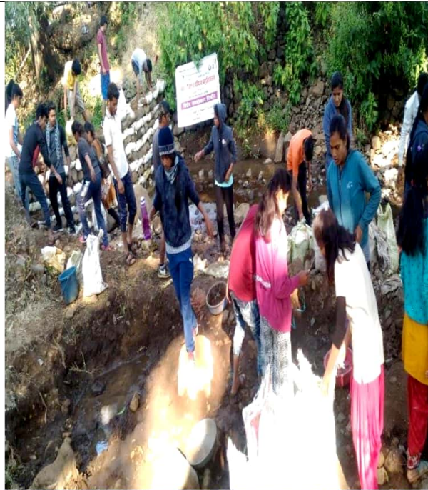
Dam Construction 21/12/2018 to 28/12/2018
