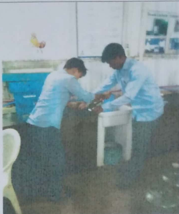
Doing maintenance Work
