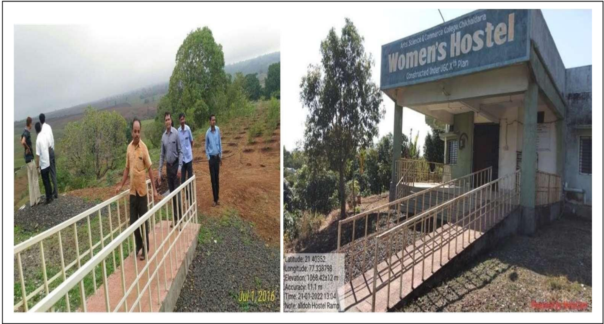
Women's Hostel Ramp
