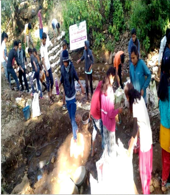
Dam Construction 21/12/2018 to 28/12/2018
