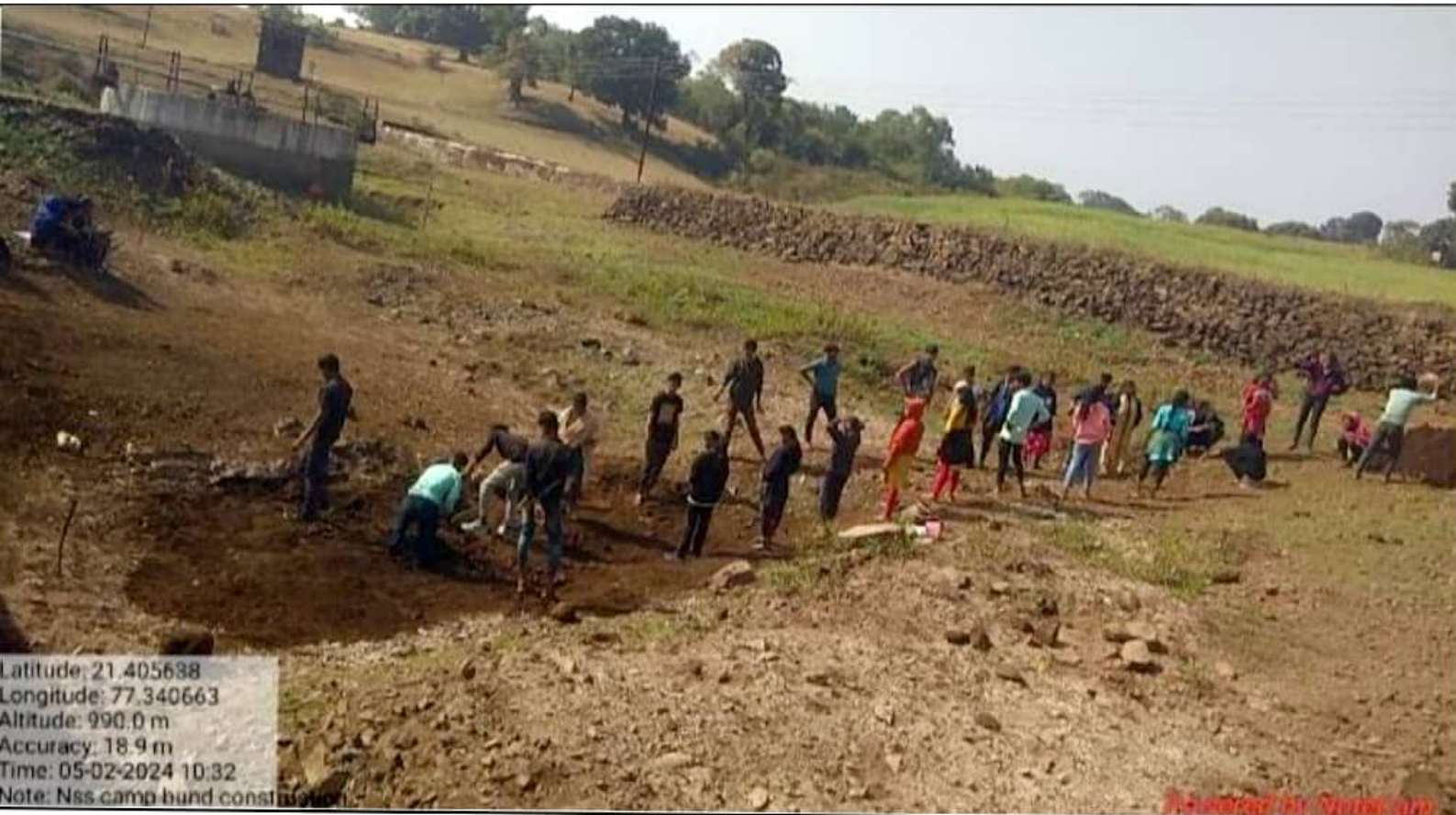
Students building the bund
