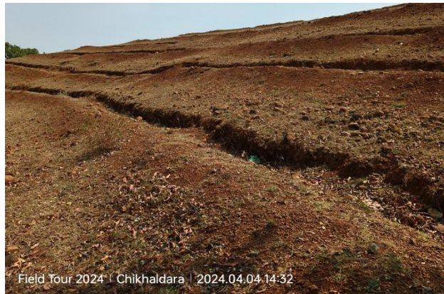
Rainwater harvesting structure viz., Tranches
